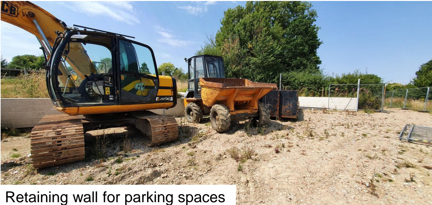
Retaining wall for parking spaces
