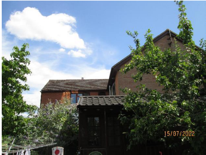
View from Adjacent Dwelling to West
